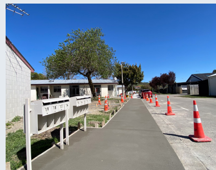
New paths and watermain repairs at Maurice Hayes
