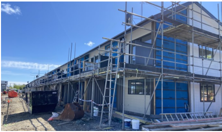
Gowerton Place is nearing completion.
